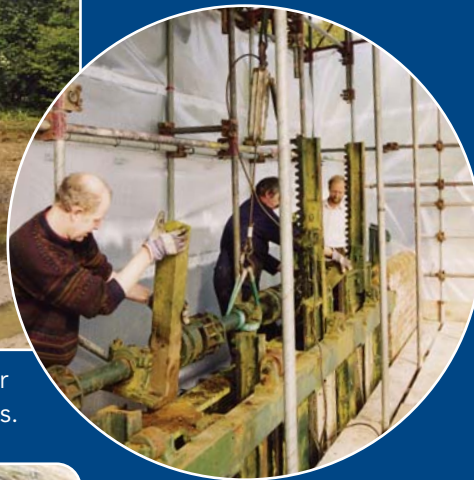
The original gearing proved to be badly damaged. New gears with improved ratios were manufactured and installed by Cast Iron Welding Services.
