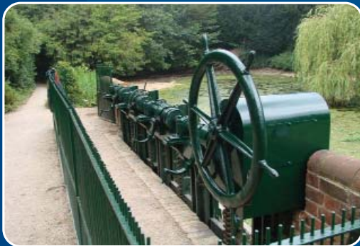
Completed sluice gates with restored mechanism and guards.
