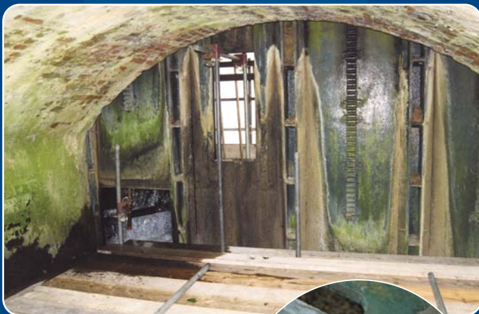
The underside of the bridge showing the scaffolding in place ready for the removal of the sluice gate mechanism.
