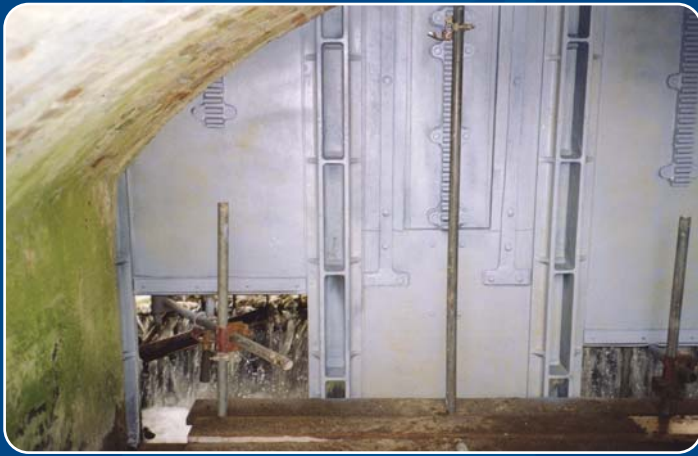
Re-fitted sluice gate section viewed from inside the bridge.
