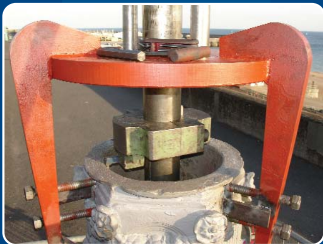
The reaming tool gets to work.
