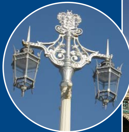
The finished job, the restored and re-painted lamp standards.
