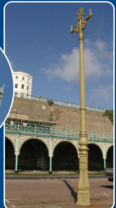
The finished job, the restored and re-painted lamp standards.
