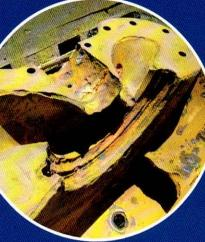
One of seven high-lift seawater pump housings with extensive internal erosion to both wear ring and stuffing box locations.
